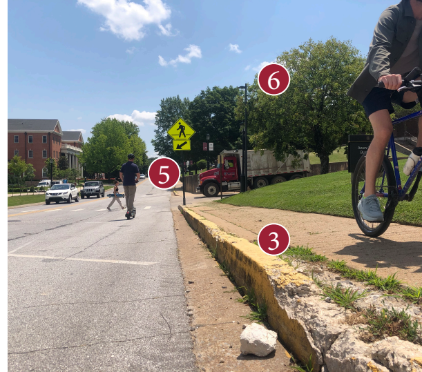
Figure 2. A broken curb on Maple St.
