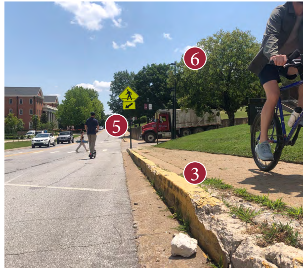
Figure 4. A broken curb on Maple St.
