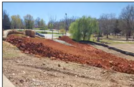
Fig 4 West bioswale being installed. Photo taken April 8, 2016. (Photo by Joanna Mentzer)
