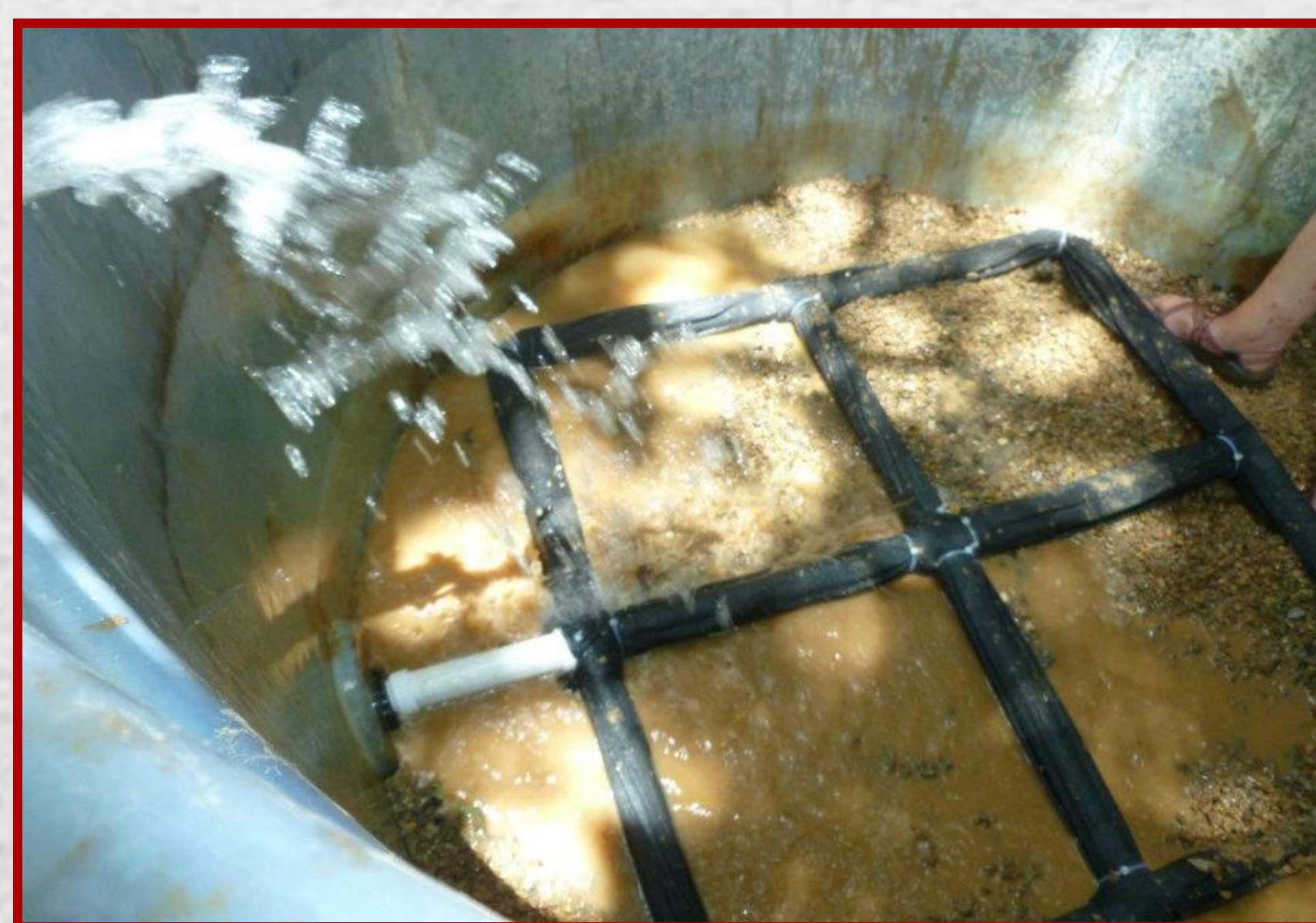
Fig. 2 Newly installed PVC filter
