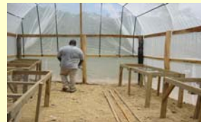
Inside the house with the completed seedling tables
