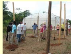
First day of work at ANRI constructing the support posts.
